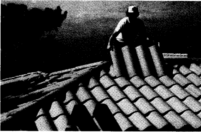
Photo 7 Fiber cement simulating clay or concrete tile.
