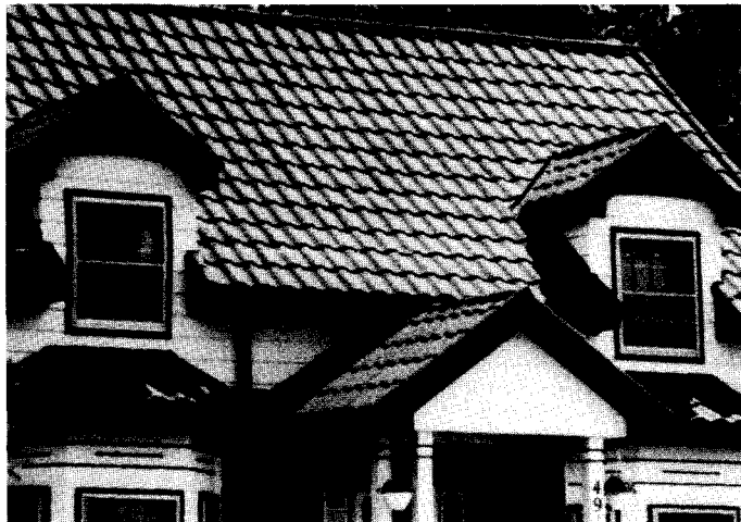
Photo 3 Metal simulating tile.
