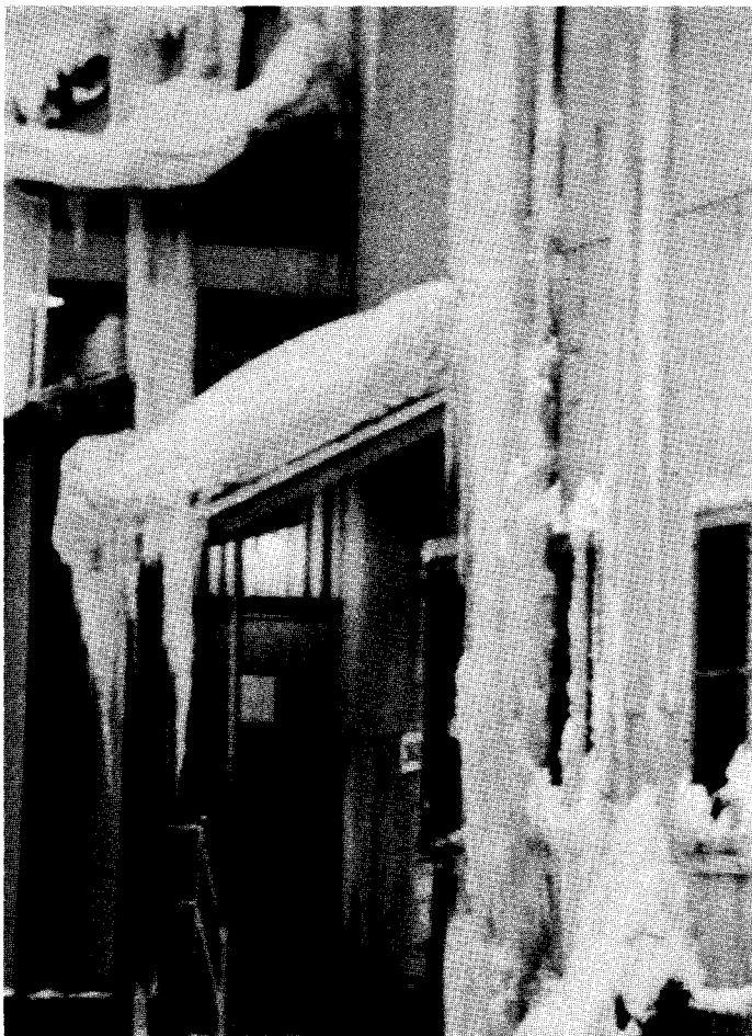
Figure 4 Ice dams and wall icings on a poorly insulated building in Fairbanks, Alaska, with a hot metal roof.
