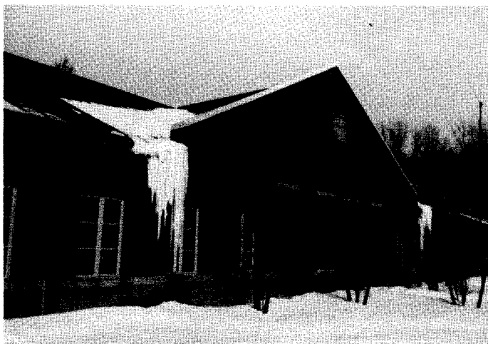
Figure 8 Large ice dams are forming at the bottom of valleys on several roofs at Ft. Drum in upstate New York.
