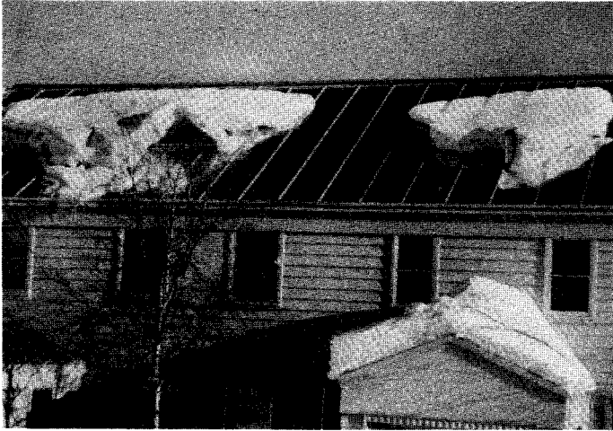
Figure 13 A small obstruction on a roof can hold back a wedge of snow.
