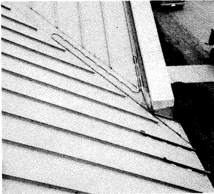
Figure 9 One of several heating cable systems being evaluated at Ft. Drum.
