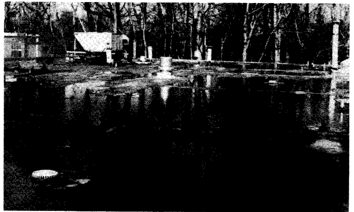
Figure 3 Example of a roof that had extensive ponding.
