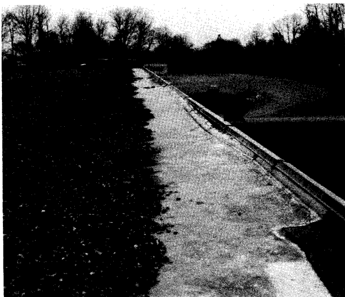
Figure 10 Shrinkage of an unreinforced ballasted PVC roof system: the ballast has moved inward away from the parapet by a few feet. Also, the exhaust pipes have been slightly pulled over, and a portion of the base flashing has pulled away from the parapet (see arrow). These conditions are potential early warning signs of shattering.
