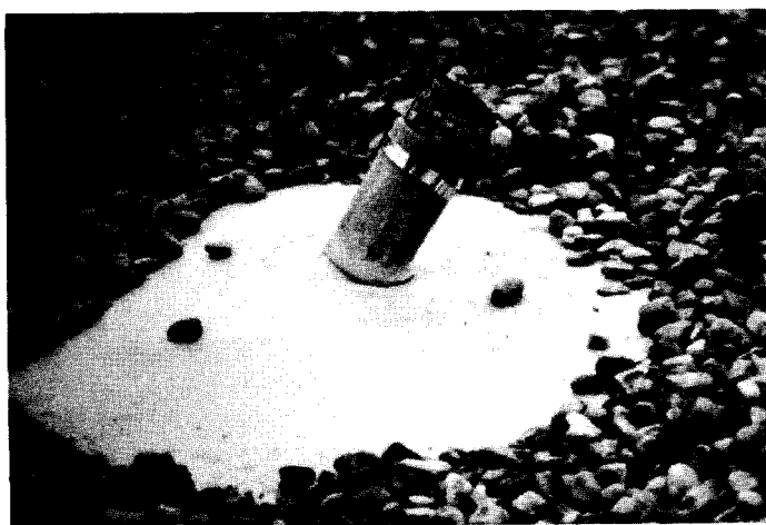
Figure 11 Shrinkage of an unreinforced ballasted PVC roof system has resulted in displacement of this plumbing vent. This too, is a potential early warning sign of shattering.
