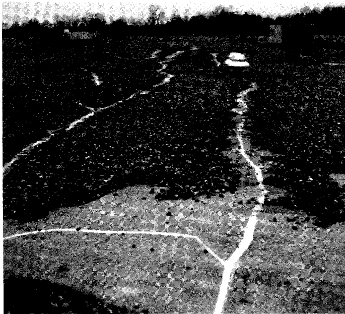
Figure 2 General view of a shattered ballasted unreinforced PVC roof system.
