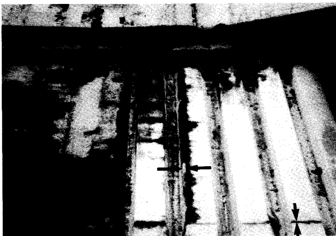
Figure 7 Close-up view of Figure 4 (phenolic "I", but in opposite direction). The galvanized deck is on the right—the dark areas are red rust (see Figure 10). Notice the enhanced corrosion that occurred at insulation side and end joints (see arrow). The prime painted deck is on the left—the entire surface is very corroded. The light colored areas on the left area are where the facer stuck to the deck.
