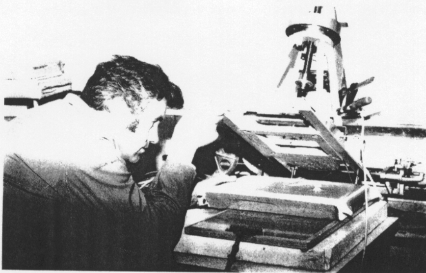
Figure 2 - Mounting of test specimen.
