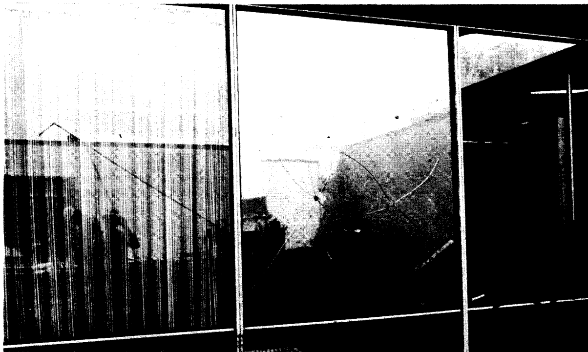
FIGURE 8 — EVIDENCE OF MISSILE IMPACTS ON GLASS WINDOWS NEAR GRAVEL SURFACED ROOFS
