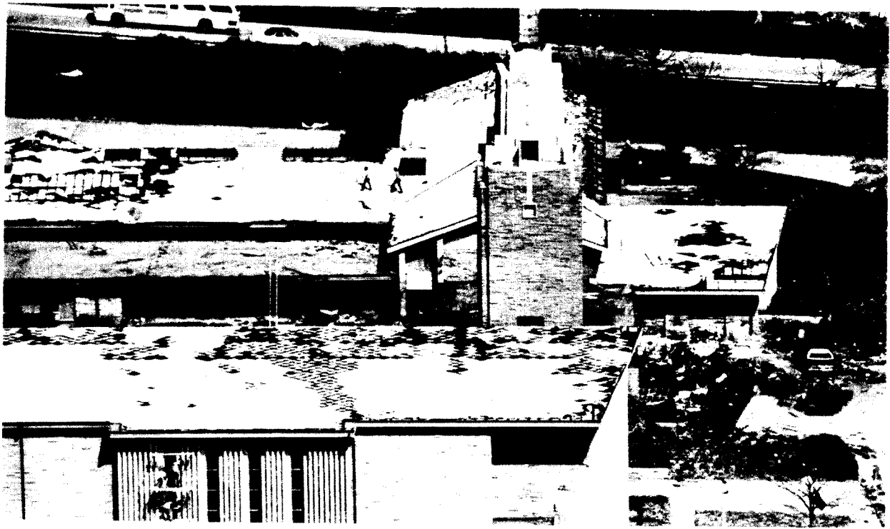
a. Relatively large pressures at roof corners, eaves, and ridges often initiate peeling types of failures
