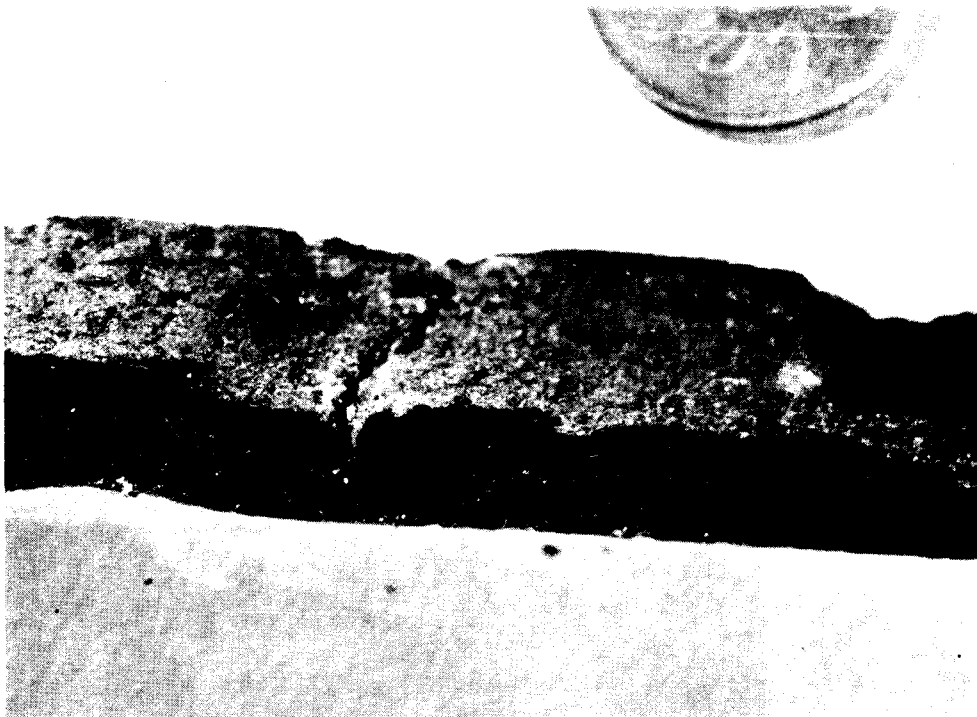
FIGURE 1 - SPLIT IN UPPER SURFACE OF MEMBRANE AND OVER JOINT IN INSULATION (NOT SHOWN). NOTE SLIGHT RIDGE (CASE STUDY 2.1.2)
