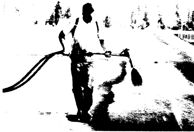
FIGURE 2 - APPLYING THE GLAS-SHIELD SYSTEM OVER THE PREPARED SURFACES.
