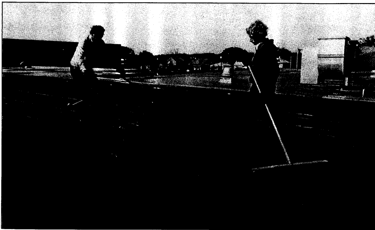
Figure 27 Application of 3-ply glass felt membrane
