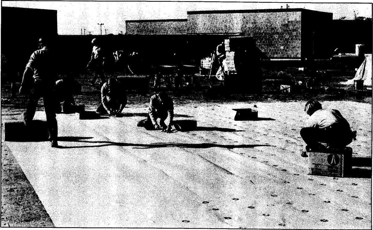
Figure 22 Covering large area with foil water seal
