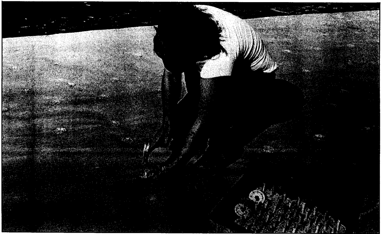
Figure 21 Close view of nailing and pre-assembly of nails and discs
