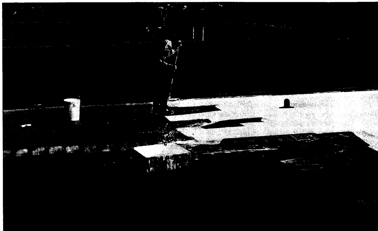
Figure 31 Application of white coating over aluminum for maximum reduction of solar exposure and heat
