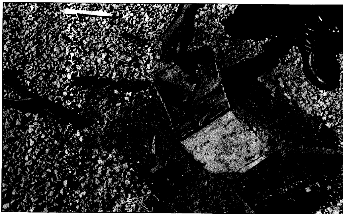
Figure 11 Riverview cut 1984: membrane dry, foil in good condition
