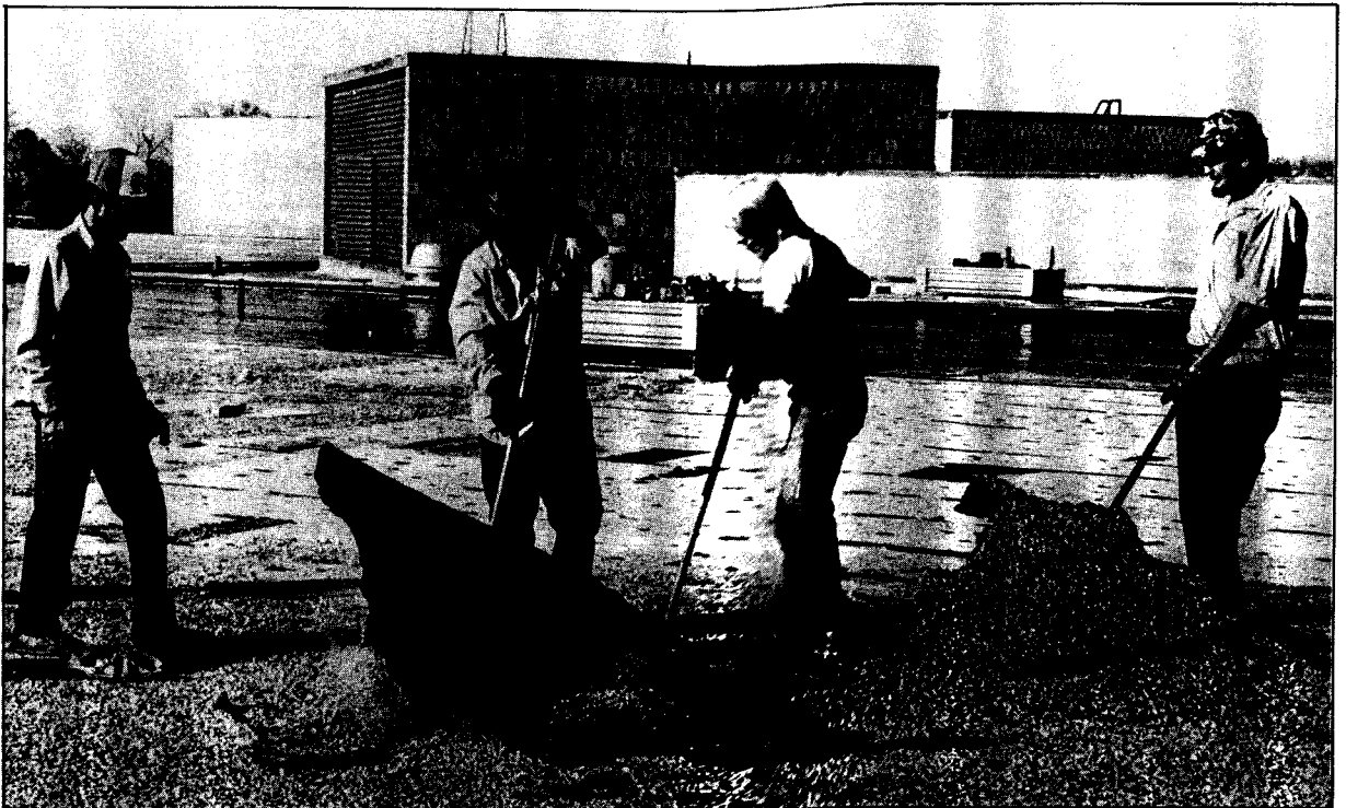
Figure 17 Tear-off of original built-up roof from wet deck
