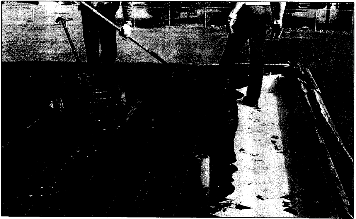
Figure 24 Mopping No. 15 felt over water seal as temporary roof ready for insulation
