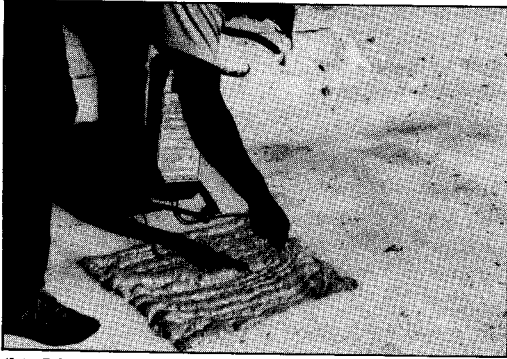
(b) PUF is patched with canned foam.
