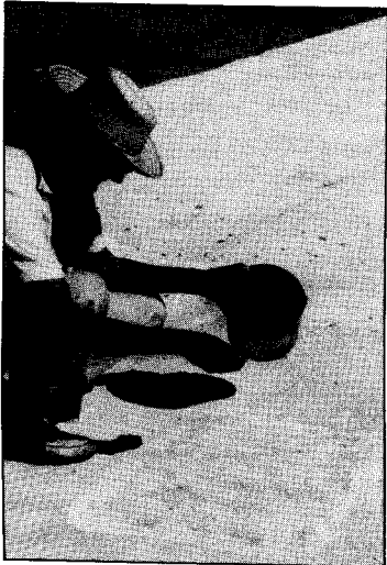
Figure 1 Patching polyurethane foam (PUF) roofs with canned foam or with foam boardstock
