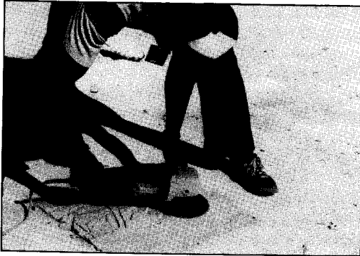
(c) Rough foam surface is smoothed with a disc sander.
