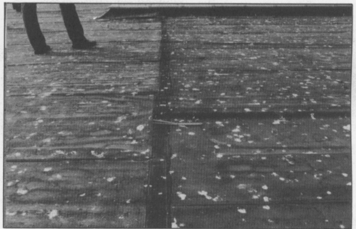
Figure 4 Shrinkage and wrinkling of the Case 2 top layer
