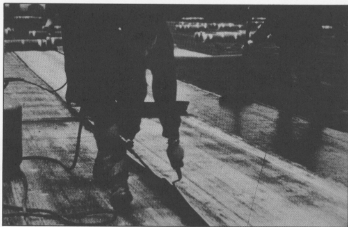
Figure 10 Application of the APP modified bitumen rolls with cold mastic in Case 6
