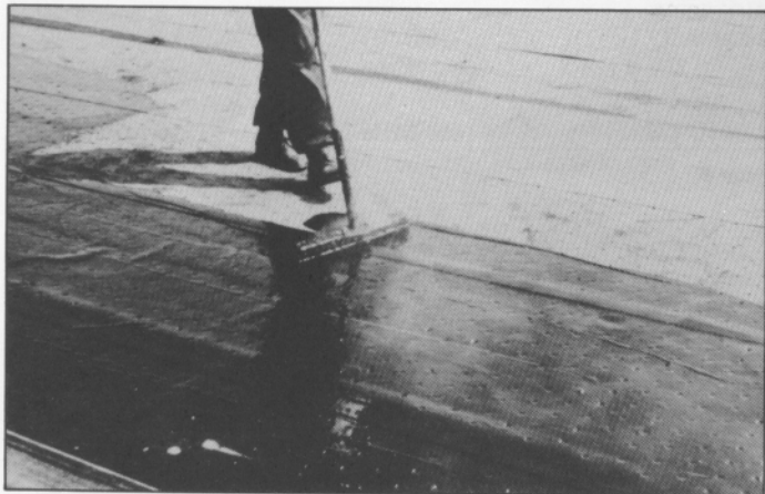
Figure 7 Installation of Case 4 floating coat
