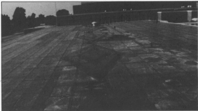
Photo 9 A completed, dead level roof—black PIB
