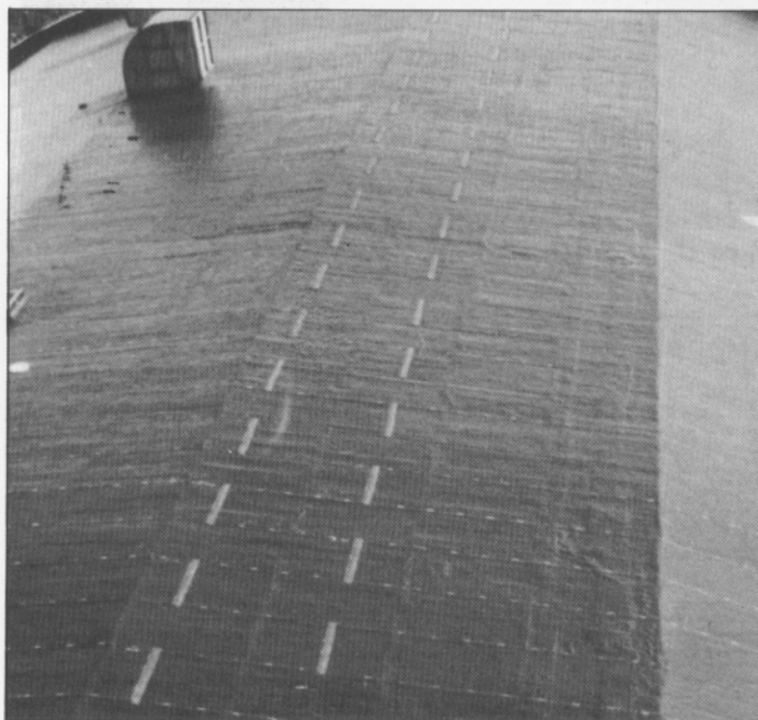
Photo 8 A completed, sloped roof—black PIB
