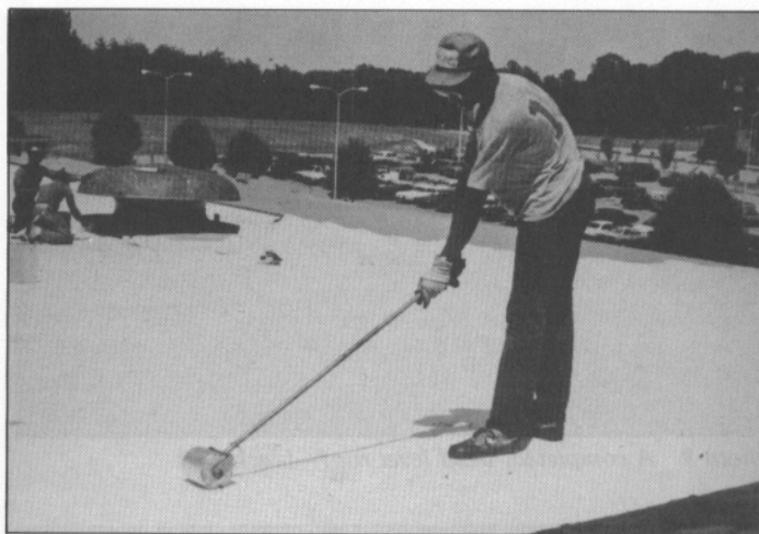
Photo 6 Rolling the seam firmly with a long handled, 35-lb. roller
