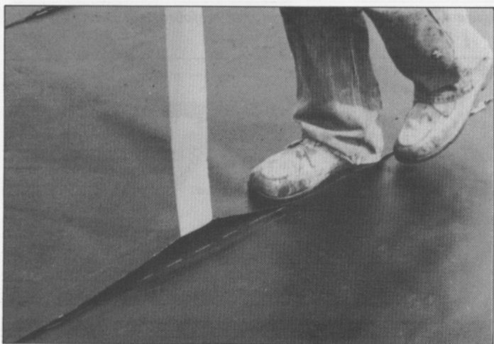
Photo 5 Removing the seam release paper strip and trodding the seam down
