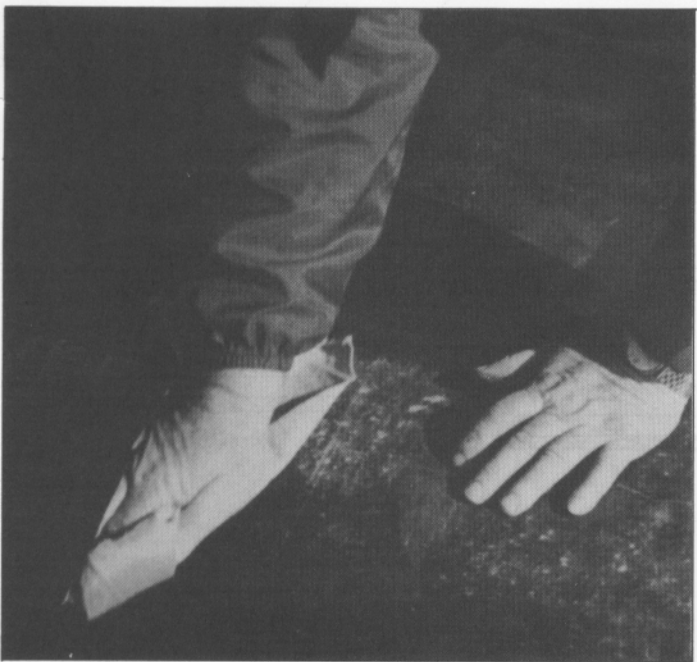
Photo 4 Cleaning the seam area with PIB solvent agent
