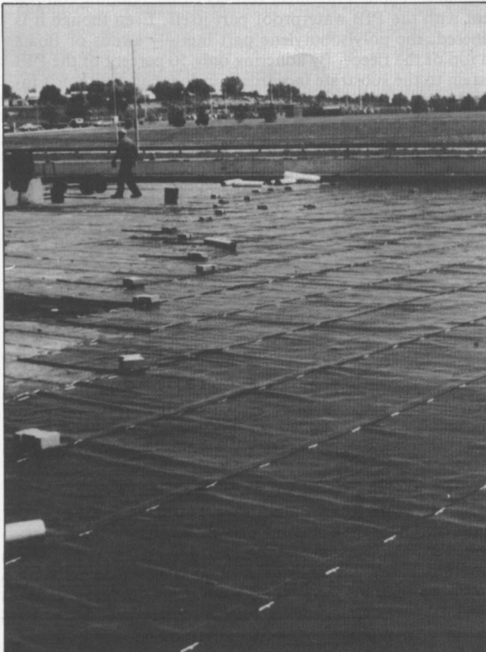
Photo 1 Laying out the PIB membrane—2" seam overlap, controlled by alignment markers
