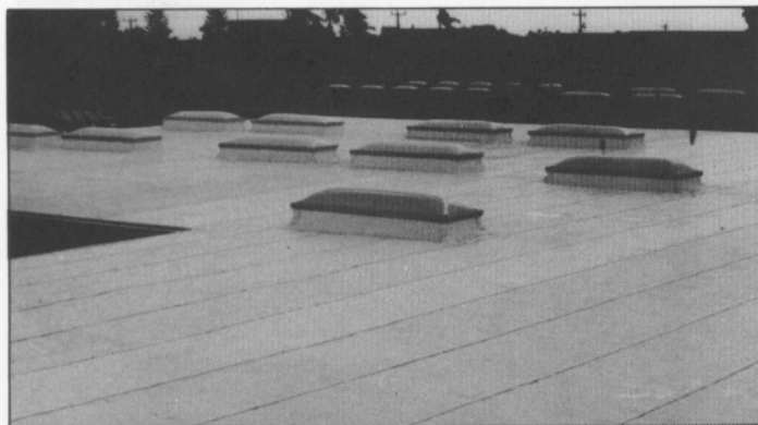
Photo 10 A completed, dead level roof—white PIB
