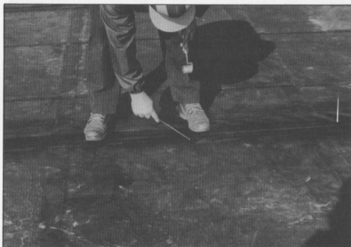
Photo 7 Controlling the seam with a needle probe
