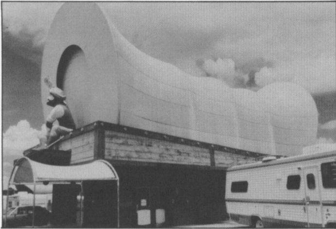
Figure 6 Wagon Ho Restaurant roof has endured the highest ultraviolet concentrations in the United States for more than 16 years without loss of structural integrity
