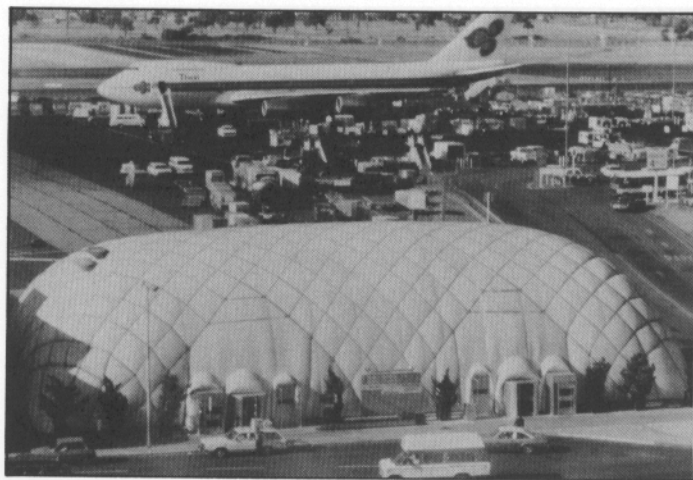
Figure 2 Los Angeles International Airport. This is one of three air-supported structures that were used by the U.S. Customs Bureau until permanent structures could be erected.
