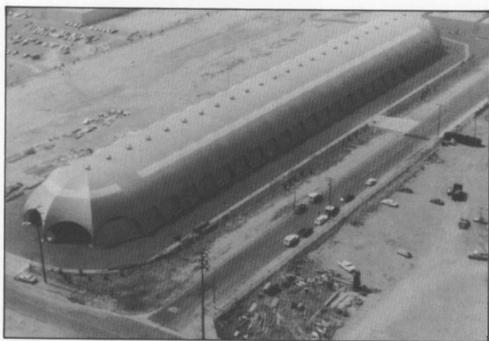
Figure 1 Garden State Paper Company. This 100,000-square-foot tension membrane structure has more than seven miles of seams under a constant tension of 60 pounds per foot. The membrane is exposed daily to high concentrations of atmospheric pollutants.
