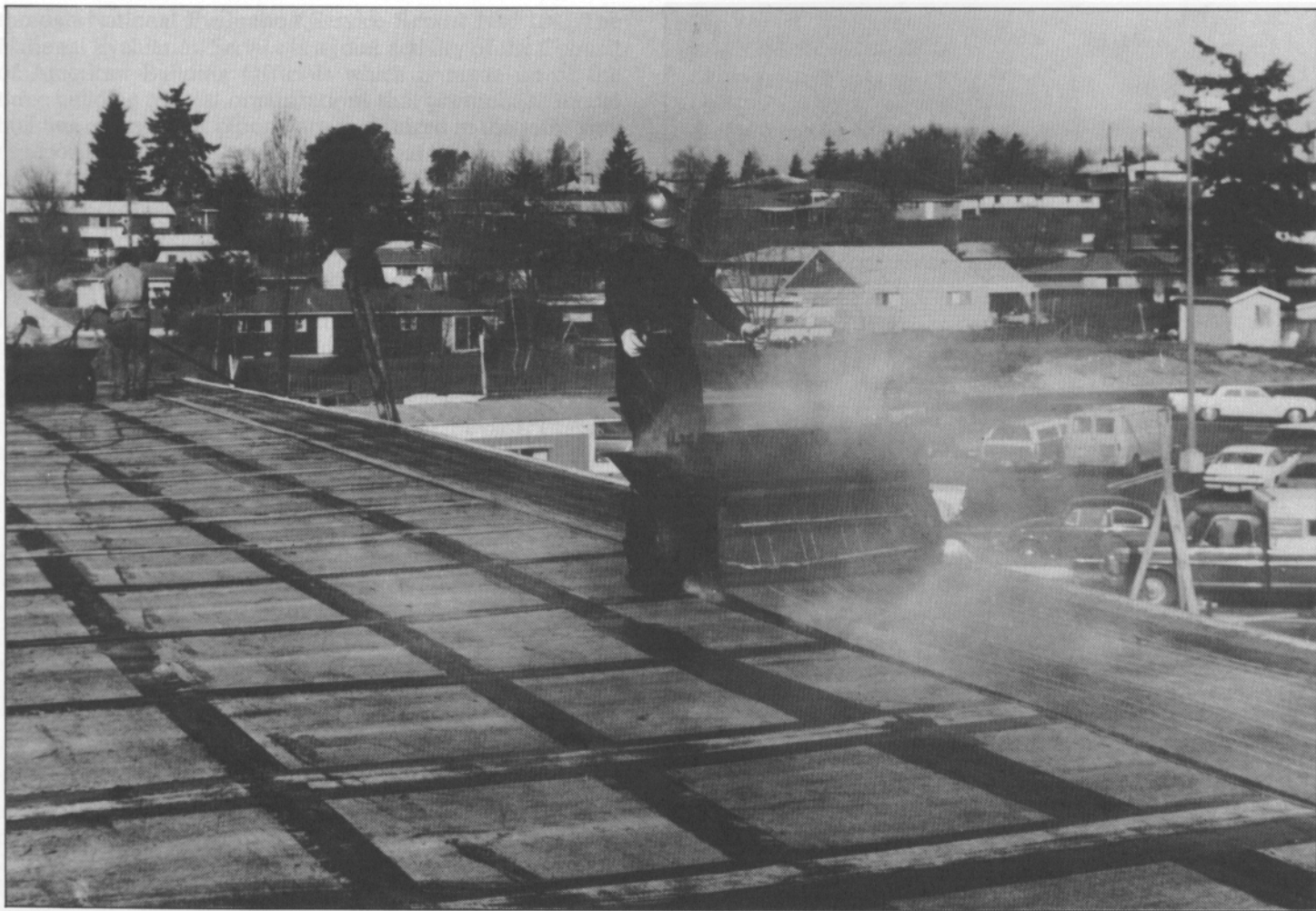
Figure 3 Roofing felt layer in operation
