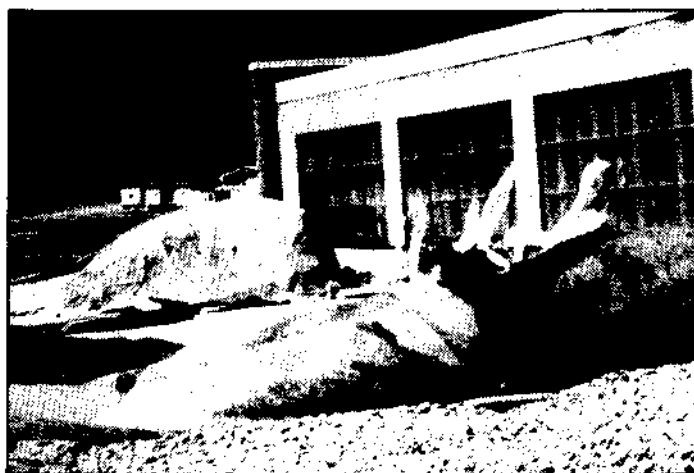
Figure 3 Taken during fatal wind, photo above shows critical configurations of ballasted EPDM. Far balloon is 5'4" high as wind speed increases from 147 mph. Note ballast dam in foreground.
