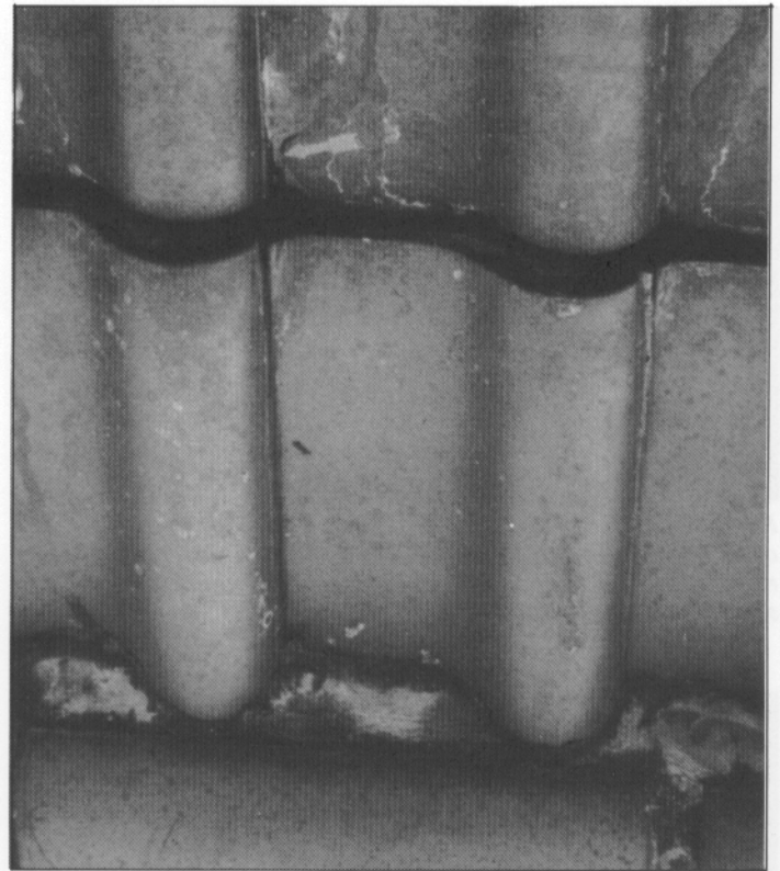
Photo 3 View of the roof ridge. A) Humidity penetration of the mortar due to condensation. B) As a result of the low outdoor temperatures (-10), the condensation which has settled between the roof tiles has frozen on the lower side of the overlaps arranged lengthways (ice has formed) (see arrows indicating the spot).
