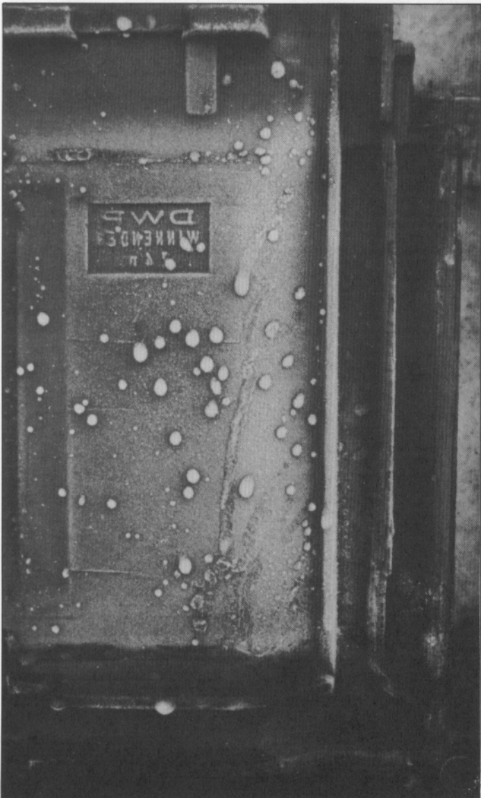
Photo 6 Detailed view of the lower portion of a roofing tile. Frozen condensation humidity.
