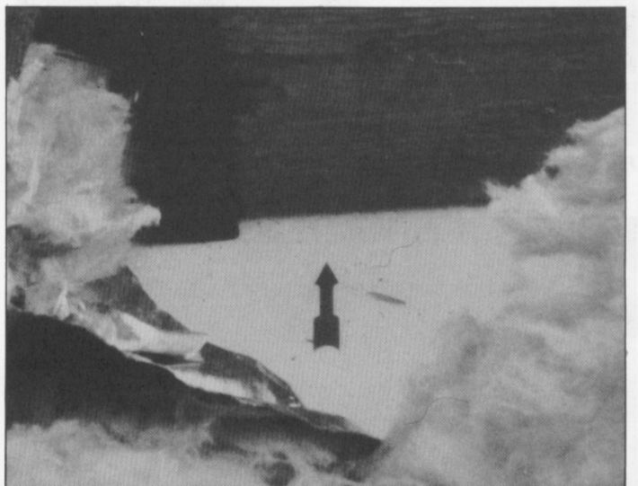
Photo 9 Complete view of the construction layers, seen from the outside looking towards the inside. The arrow indicates the thermal insulating layer on the side towards the room, consisting of polystyrene particle-foam. The rafter sides are heavily impregnated with humidity on the upper surface. (Depth of penetration of humidity, up to 5mm on the average).
