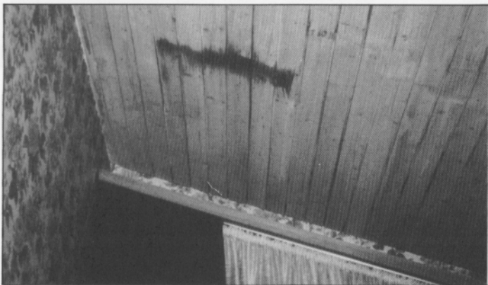
Photo 2 Inner view—living room. Wood paneling of the ceiling discolored through condensation.
