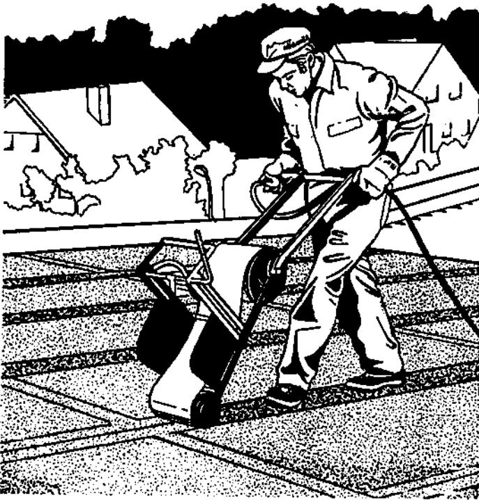
Figure 11 Special joint strips are applied by a welding technique
