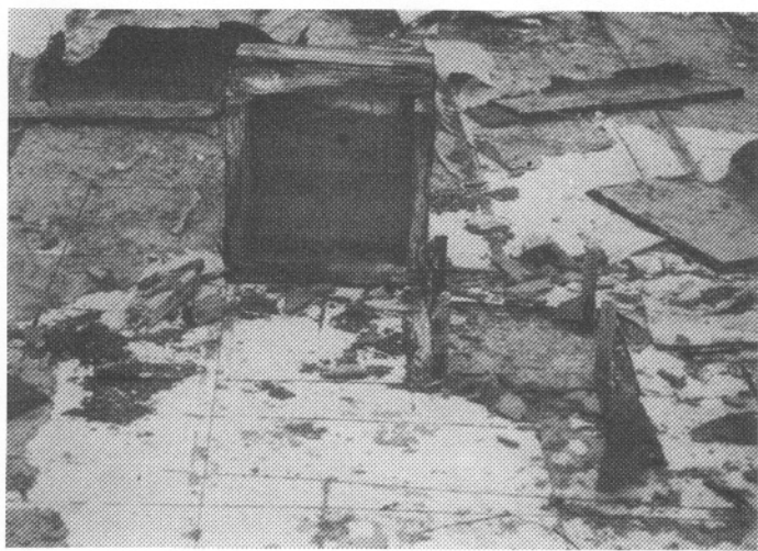
Figure 11 Wood curb built over a steel column.
