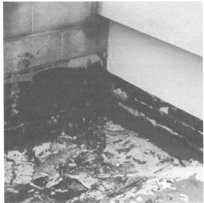
Figure 9 Moisture deterioration of an unprotected fiber cant.
