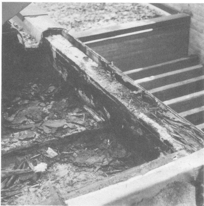
Figure 10 Deterioration of a wood blocking on an exterior wall.
