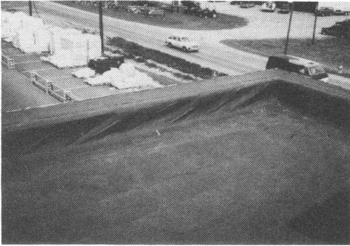
Figure 1 Wrinkling and/or tearing of base flashings (wrinkles highlighted with white chalk).
