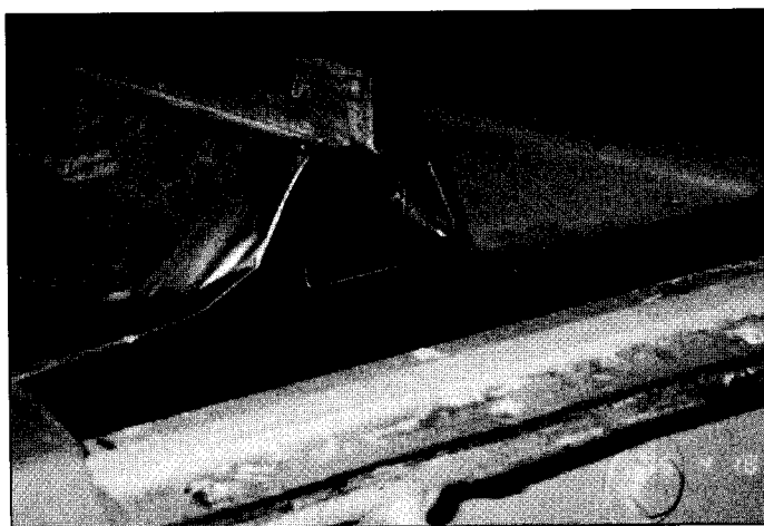
Figure 1. Rolled seam over purlin showing clip fastener.
