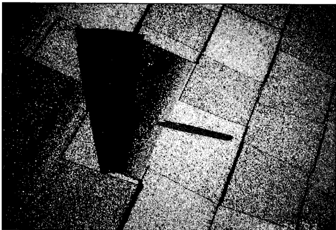
Photo 13. A staple (near the end of the pen) drove all of the way through the shingle.
