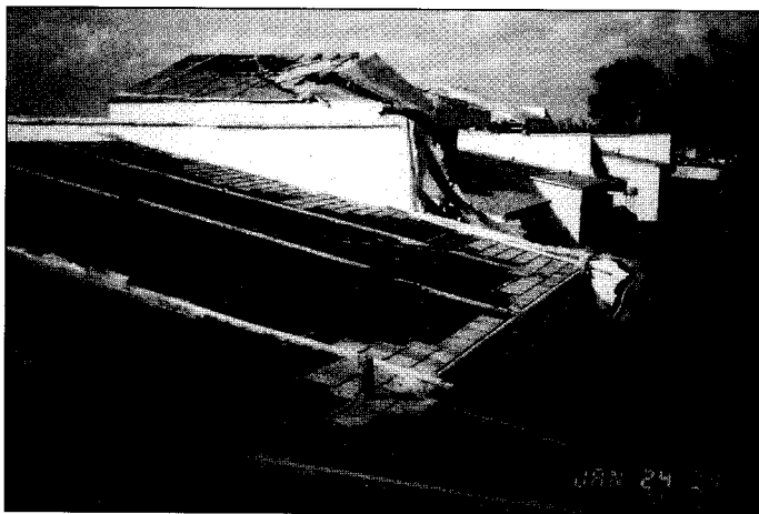
Photo 11. Some underlayment was lost (bottom center of the photo). The wood strips running up the roof had been placed to hold down polyethylene sheeting, which was no longer in place when this roof was observed in January 1993. On one of the other roof areas of this building, it appeared that wind-blown debris may have initiated the shingle failure.
