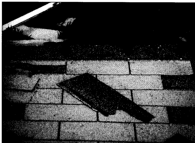
Photo 17. This section of plywood decking blew off. The shingles were each attached with four nails, which were located in the self-seal strip (see arrows).
