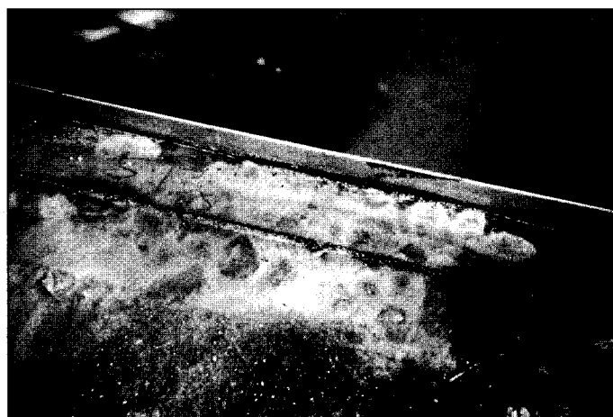
Photo 7. Roof S13: The field sheet is fastened with roofing nails that were also used to attach the metal edge flashing. The nails were spaced at 5 in., 5 in. and 4 in. (125, 125 and 100 mm). The field sheet turned down at the wall and was fastened by the continuous cleat fasteners. As the field sheet moved inward, the originally uncured flashing was stretched and torn.
