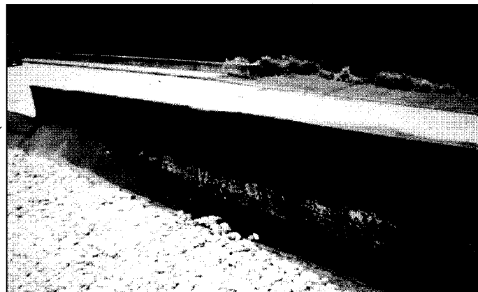
Photo 1. After the field sheet was torn at the metal batten, the originally uncured flashing over the batten stretched and tore. (Georgia)
