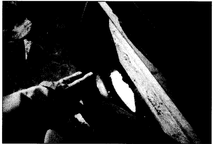
Photo 2. Roof S5: The field sheet was attached to a CMU wall with wood battens that were fastened with plastic sleeves/drive pins, spaced at 12 in., 11½ in. and 9½ in. (305, 290 and 240 mm). The field sheet tore and pulled out from under the batten at the fastener locations. The originally uncured flashing over the batten was then stretched and torn. At other locations, the fasteners pulled out of the wall and the batten moved inward approximately 6 in. (150 mm).
