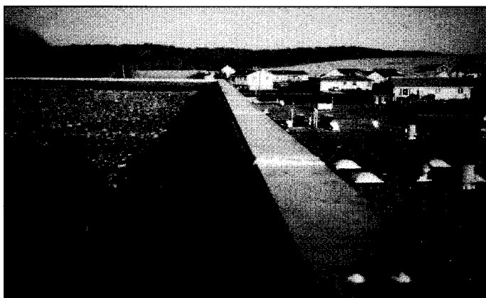
Photo 4. Roof S9: Along most of this parapet, the wood batten fasteners pulled out of the brick. In some locations, patches had been placed where the ends of the battens had punctured the flashing.
