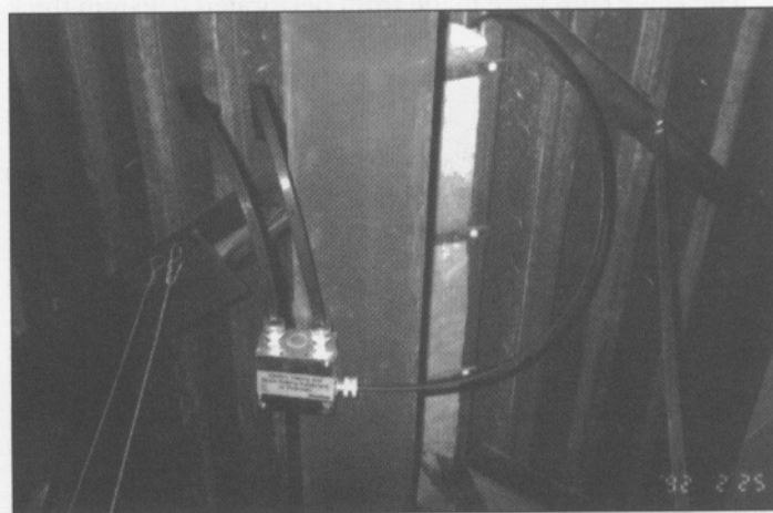
Figure 5. System with high output heater installed below the metal roof in a valley.
