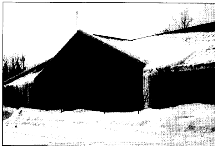
Figure 2. Large ice dams and icicles form where the gable parapet ends at the bottom of valleys.
