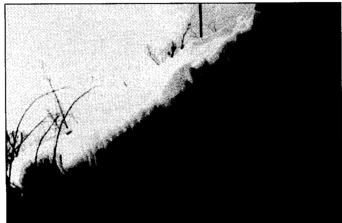
Figure 15. Icings forming on a creeping, overhanging mass of snow and ice bypass the heated fascia on this building. Note exposed heaters at near end of fascia.
