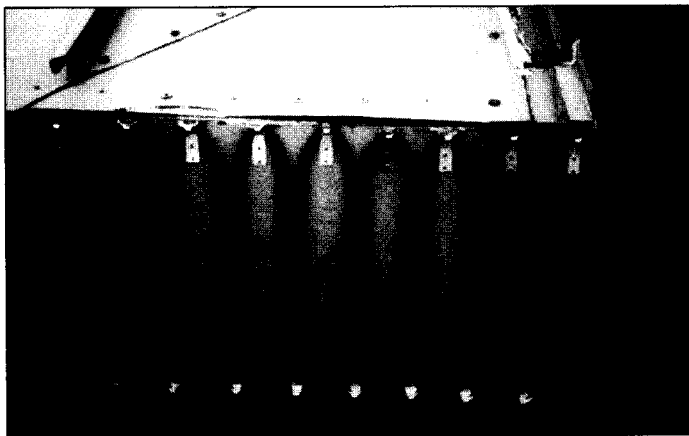
Figure 12. Heater looped over butterfly clips mechanically attached to fascia.
