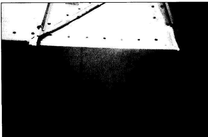
Figure 13. False closed-top fascia installed over heater shown in Figure 12. Note heated vertical baffles (water diverters) at each end.
