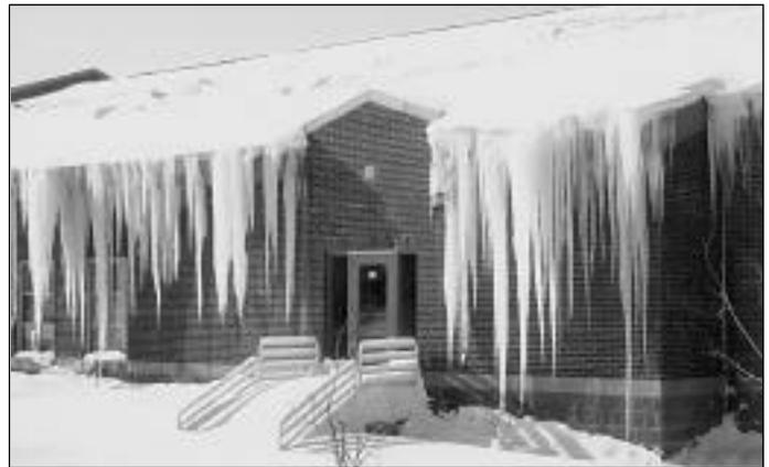
*Figure 1. Severe icings along the eaves of a poorly ventilated roof.*
