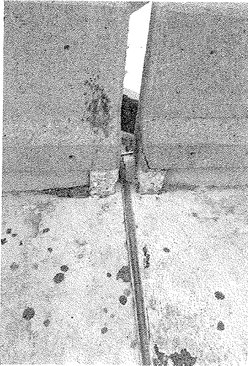
A typical friction fit joint
