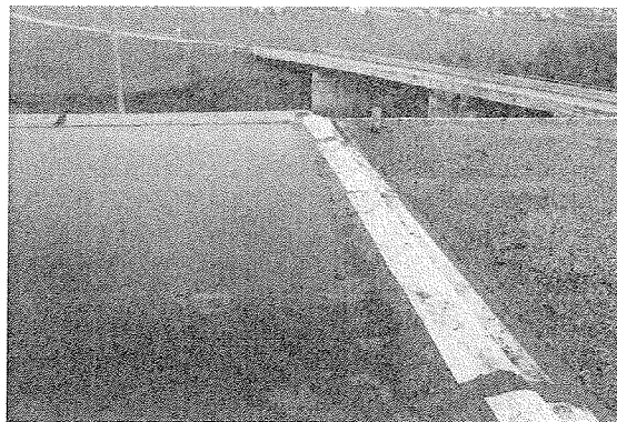
The water ponding effect of a raised expansion joint.
