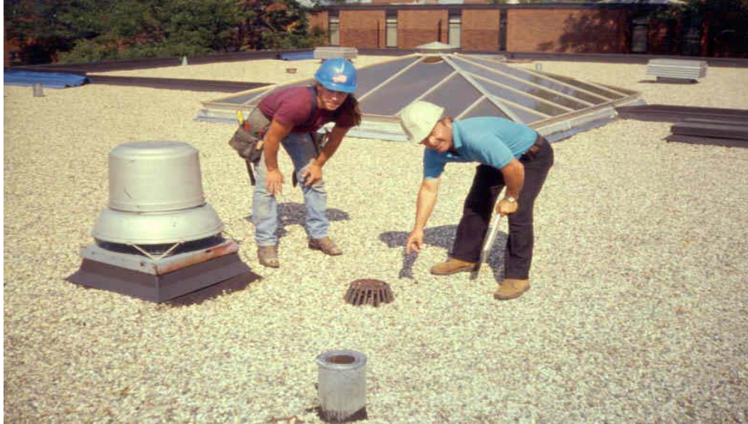
Annual Roof Survey
