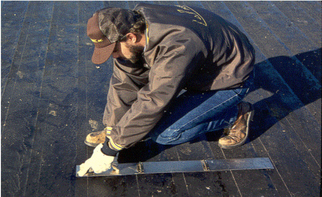
Roof Membrane Test Cut
