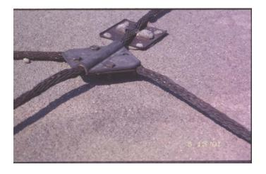
**Figure 11.** The bolts through this cross-run clamp are resting on the roof membrane. A conductor connector occurs near the top of the photo. It was attached to the membrane with sealant.
