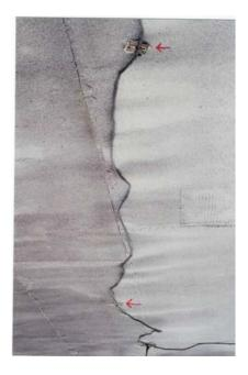
*Figure 6.* The spacing between these conductor connectors (shown by arrows near the top and bottom of the photo) greatly exceeded the 3 foot (915 mm) maximum requirement.
