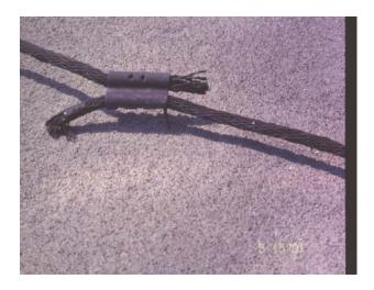
**Figure 10.** This conductor splice is upside down. One of the prongs of the splice plate was not clamped to the conductor -- the prong is resting on the roof membrane. As with the condition shown in Figure 5, the membrane is vulnerable to puncture by the frayed strands and splice prong.
