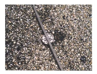
**Figure 8.** This conductor connector had been adhered in asphalt roof cement to an aggregate-surfaced BUR. Because the cement was applied to loose aggregate, the conductor could be easily moved.
