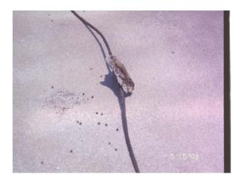
**Figure 7.** This is the upside-down base of an air terminal (the terminal rod is missing). The base had previously been adhered to a built-up membrane -- it had not been adequately cleaned and readhered to the new SPF roof.
