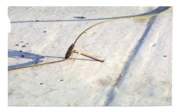
*Figure 12.* This air terminal was dislodged and whipped around during a hurricane. The single-ply membrane was punctured by the sharp tip in several locations.
