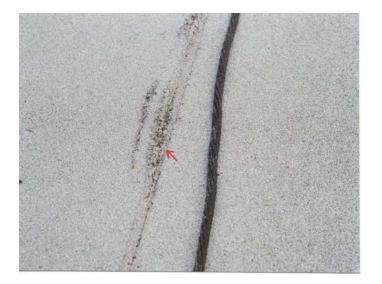
**Figure 5.** This conductor occurred on a white cap sheet in Florida. The conductor had previously been located to the left where marked by the arrow. At the previous location, the conductor had sunk into the membrane, thereby displacing the bitumen above the reinforcement.
