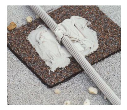
*Figure 4.* A pad of cap-sheet material was adhered to the mineral-surfaced membrane. The conductor was set in and covered with sealant.
