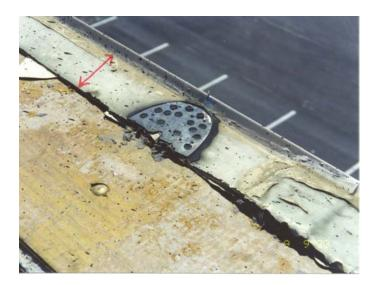
**Figure 13.** View of location where an air terminal base was adhered to an EPDM membrane. The arrows indicate the horizontal flange of the metal edge flashing. The conductor became dislodged during a hurricane. The loose conductor whipped and tore the membrane. The torn membrane was eventually lifted and peeled off the roof insulation. See Figure 14.
