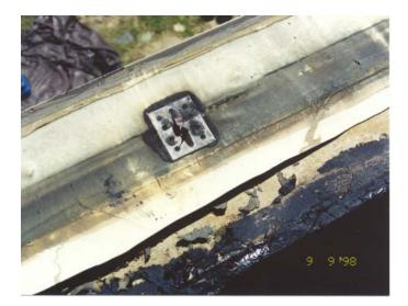
*Figure 15.* In this area, the conductor pulled out from the conductor connector. The connector was adhered to the EPDM membrane.
