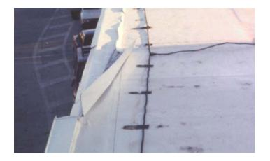
**Figure 3.** The conductors on this PVC membrane roof were attached with narrow strips of PVC sheet that were placed over the conductors and then welded to the roof membrane. In this area of the roof, the attachment strips were peeled off the roof membrane (the plane of failure occurred within the membrane, wherein the PVC matrix separated from the reinforcement).
