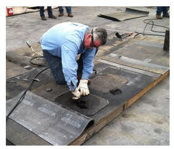
Cut a hole 18 inches from one side and 18 to 24 inches from one end in two of the three basic flat deck mockups. Use a 9-inch metal pie tin, large coffee can or an inverted galvanized steel "tall cone" flashing cut to height to simulate a roof drain opening. Secure the simulated roof drain in the hole.
