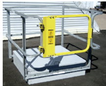
Roof hatches with permanent guardrails
