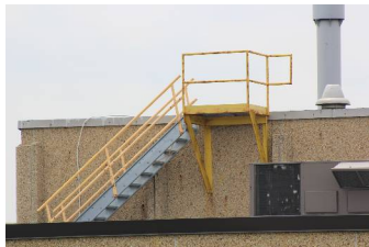
Exterior staircase and fixed ladders for roof access
