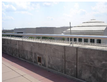
Permanent guardrail and parapet protecting rooftop terrace
