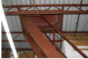
Ships ladder access to roof hatch
