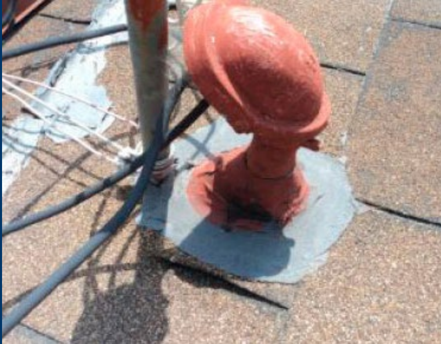
Electrical service drop on roof
