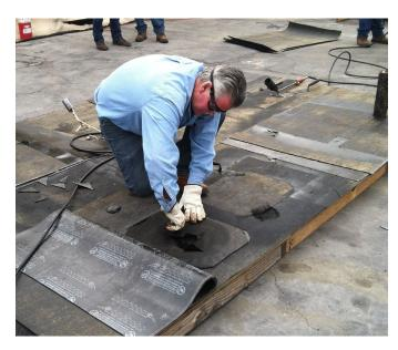
Cut a hole 18 inches from one side and 18 to 24 inches from one end in two of the three basic flat deck mockups. Use a 9-inch metal pie tin, large coffee can or an inverted galvanized steel "tall cone" flashing cut to height to simulate a roof drain opening. Secure the simulated roof drain in the hole. Basic Flashing Box Mockup
