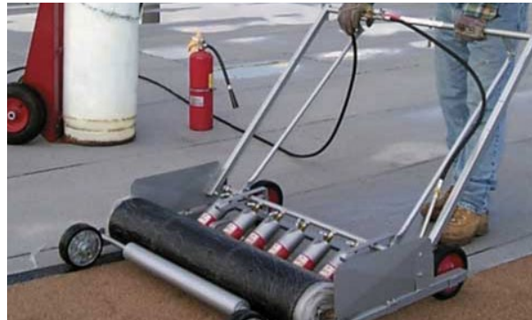
Photo 3: A roofing worker pulls a torching trolley backward.
