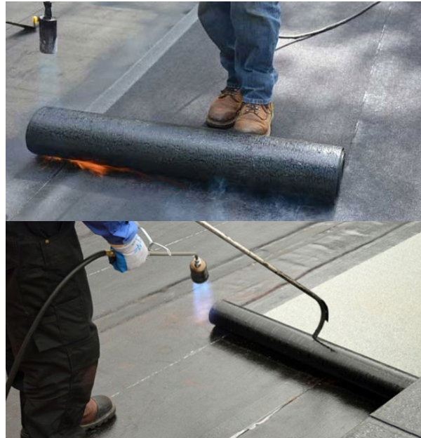
Photo 2: A roofing worker is advancing a roll of membrane.
