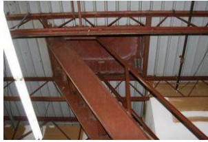
Ships ladder access to roof hatch
