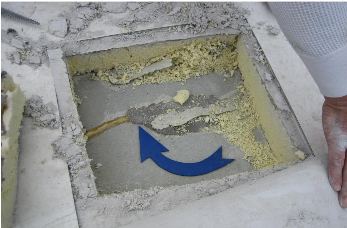
Photo 6 The photo demonstrates 3-inch single-layer insulation below the cover board in Photo 5. The moist insulation facer parted from bottom insulation facer is a typical consequences of moisture gain from new lightweight structural concrete observed in studying this type of deck construction. Wind uplift initiated discovery of problem.
