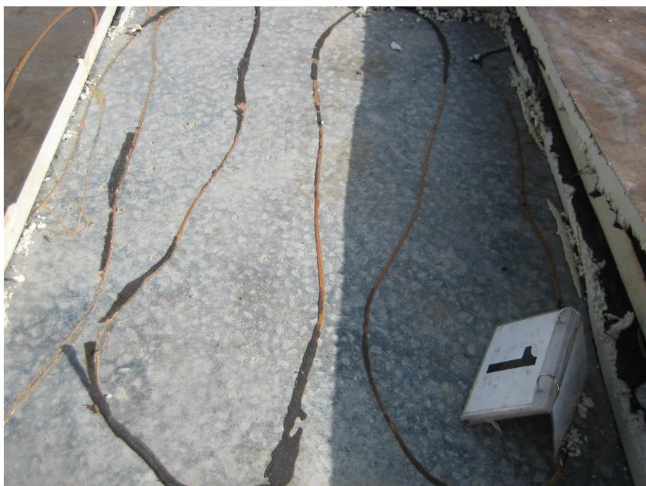
Photo 2 Bead adhesives on lightweight concrete deck show portions of insulation facer attached to adhesive; insulation boards had lifted.
