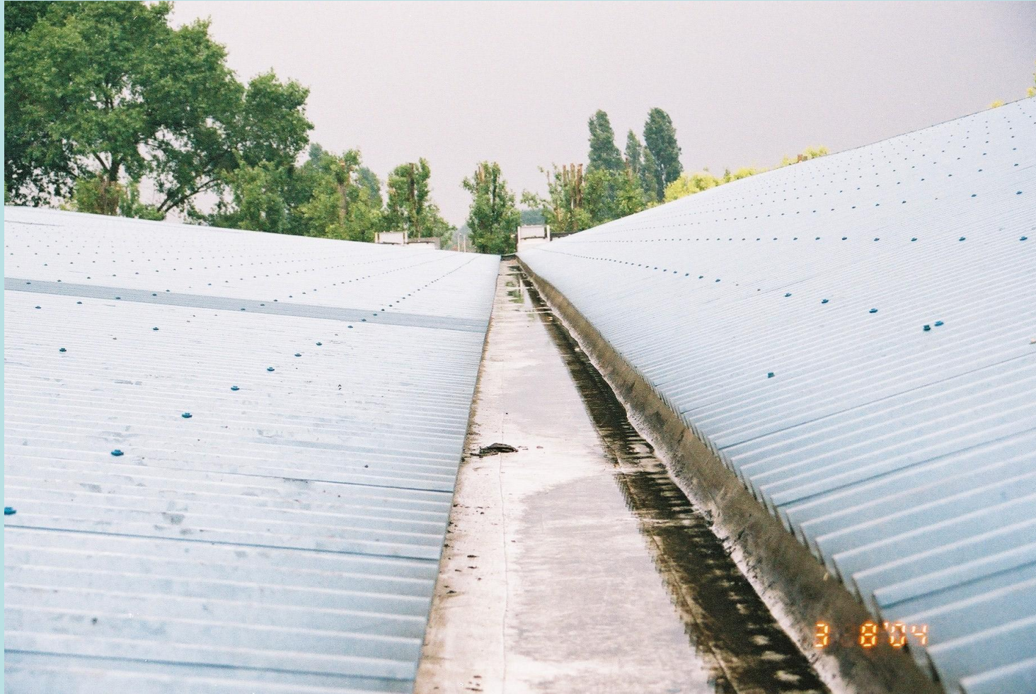
Rainwater build up in level gutters
