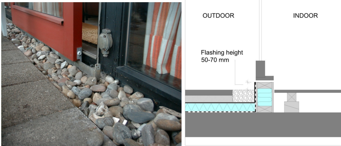
Figure 6: Example of flashings between terrace and apartment
