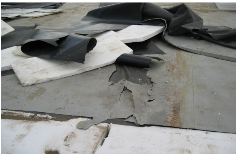
Figure 7: The loss of plasticizers was critical because it caused the membrane to shrink and become brittle.
