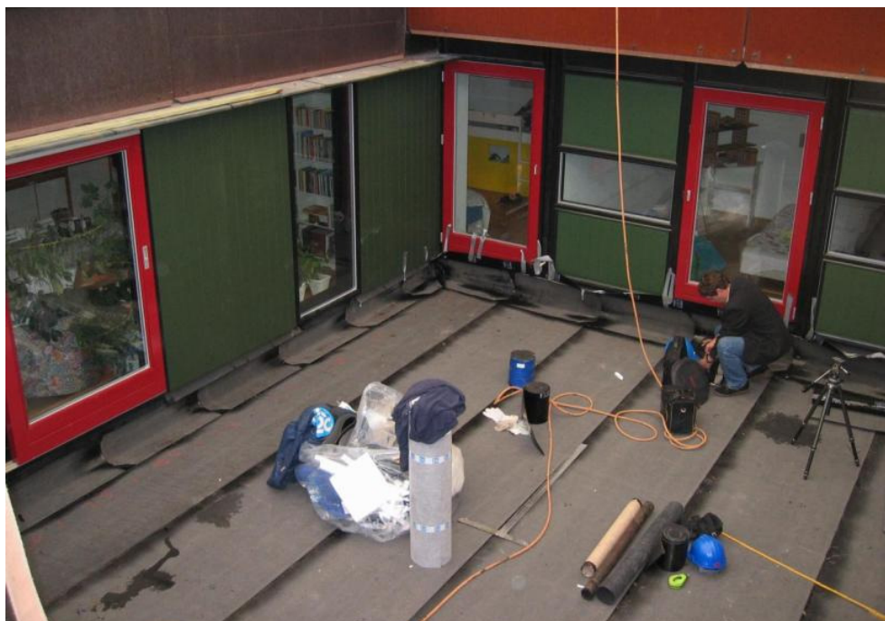
Figure 9: The membrane is installed in a roof terrace after replacing the two facades to create higher up stands.
