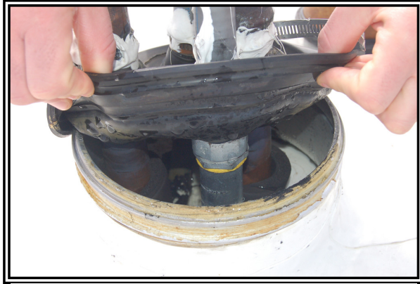
Photo 6: One of several concerns with portal type flashings is they are not sealed, allowing air movement from the interior to the EPDM cover where condensation occurs.
