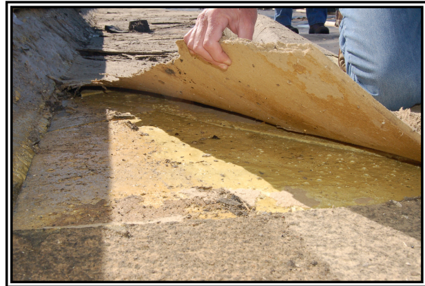
Photo 2: For spray foam adhesives to properly secure materials together, the materials need to be compressed through rolling and not rely on gravity and/or foot traffic to do so.
