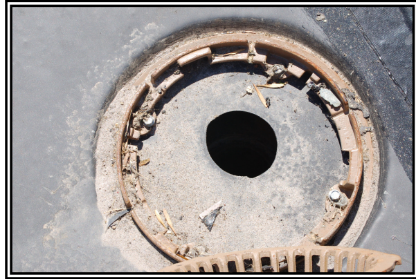
Photo 5: There is no universal contest regarding who can create the smallest opening in single plies at roof drains. Open it up to its maximum size.
