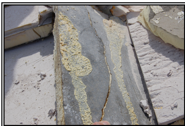
Photo 3: Bead foam adhesives must be applied to clean substrates, and the materials to be adhered must be compressed through rolling to assure a quality bond and eliminate creation of an air space between foam beads.
