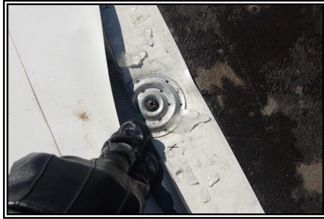
Photo 1: Ice below roof membranes, the result of condensation, is a conundrum for architects, contractors and those in the cool roof movement.
