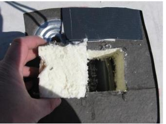
The objective was to examine roof systems using highly reflective roof membranes in heating climates by cutting into the roof systems and examining them for moisture accumulation.
