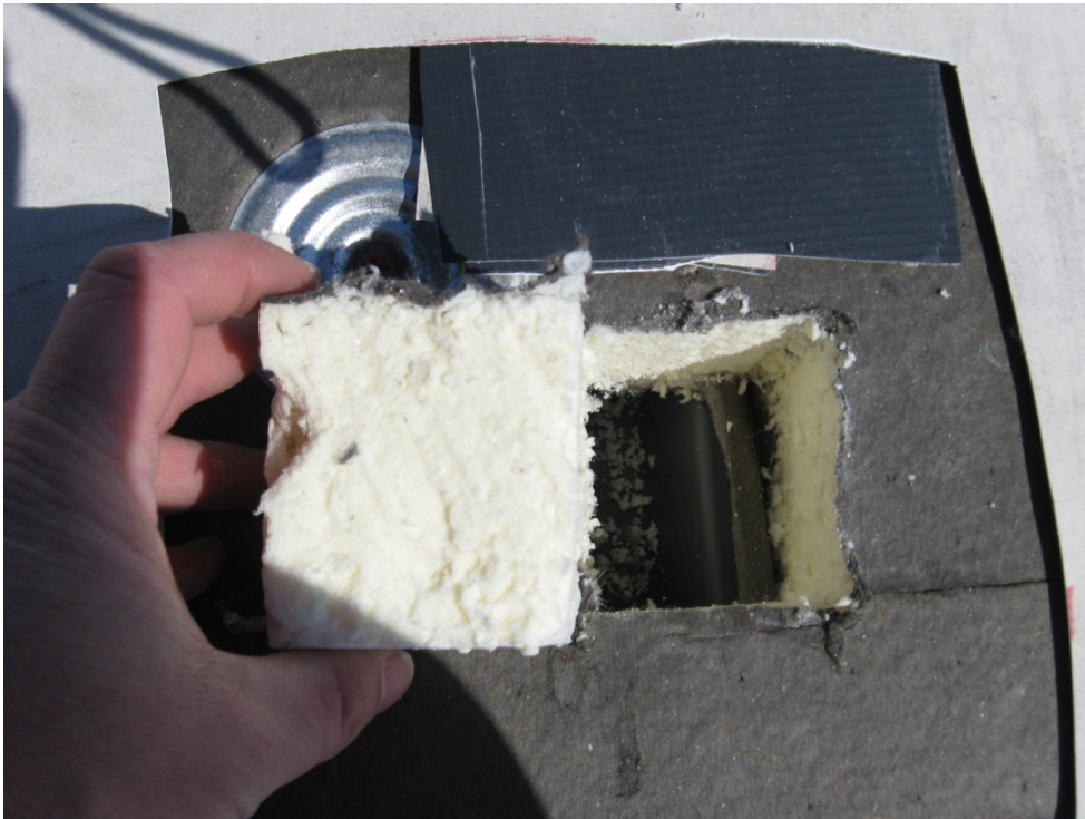
Figure 5—Example of foam test cut in Erie, Pa.
