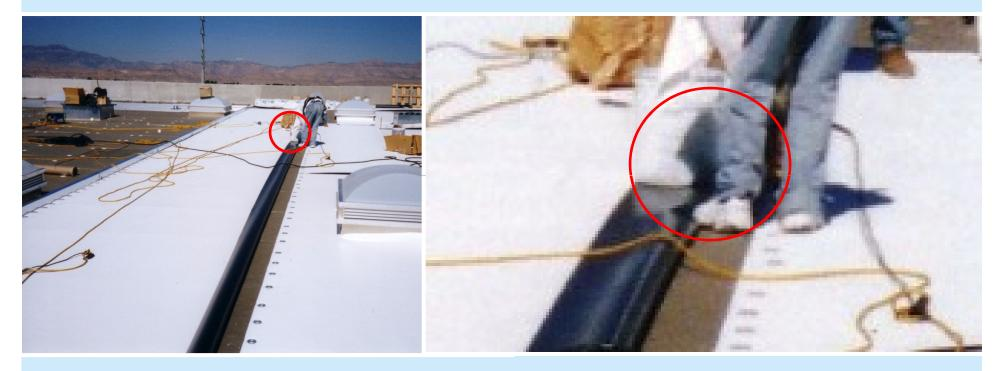
A photo from original installation of the TPO membrane in 2000. Note how the bucket and roofer's foot are hard-creasing the membrane.
