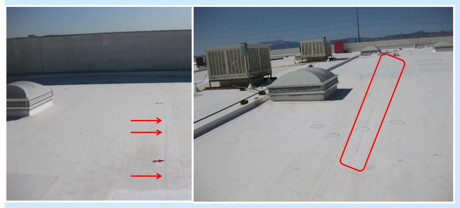
A side lap seam where creasing during installation and sun/heat load have led to cracking of the creases (2011)
