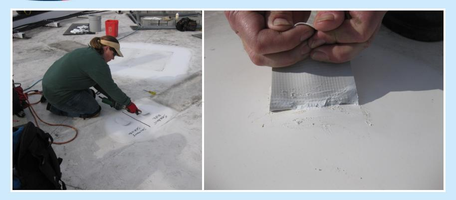
Test patches were welded on the existing membrane, then field peel tests were performed.
