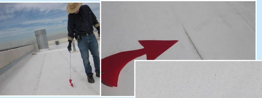
A close-up view of an isolated "crease crack"
